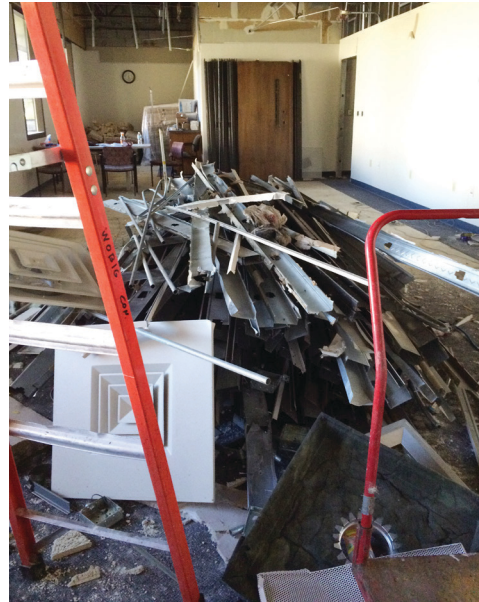
Flashback of construction progress at SCCMHA's Hancock Street building throughout 2015.
